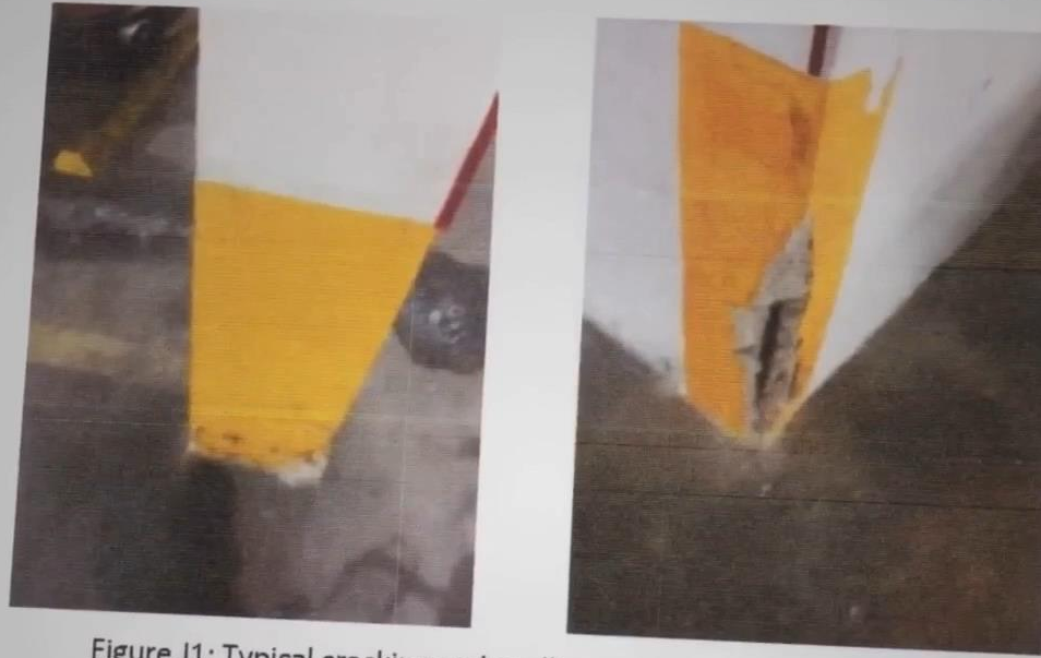
Figure J1: Typical cracking and spalling at parking garage columns
