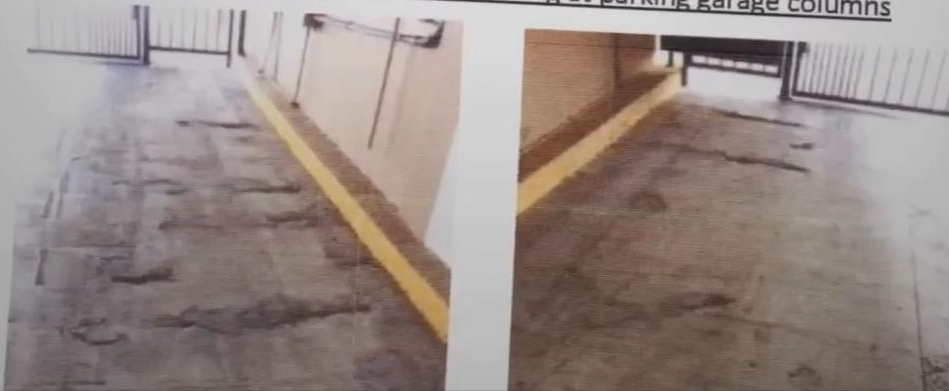
Figure J1: Typical cracking and spalling at parking garage columns
